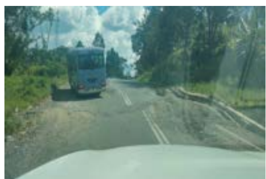
road left rippled after recent earthquake
