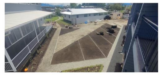
Above shows the new driveway and parking being completed by Dave & the Team using a system of Geogrid similar to used on our rural airstrips which will allow the car parking bays to all grass over in the coming months and so help soften the impact of the necessary parking.
